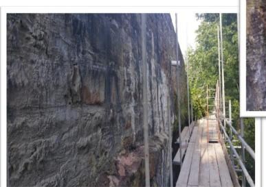
APA Concrete Repairs Ltd were the successful tenderers for the repair project with the objective of encapsulating and strengthening the existing rock face with a sprayed concrete overlay.
